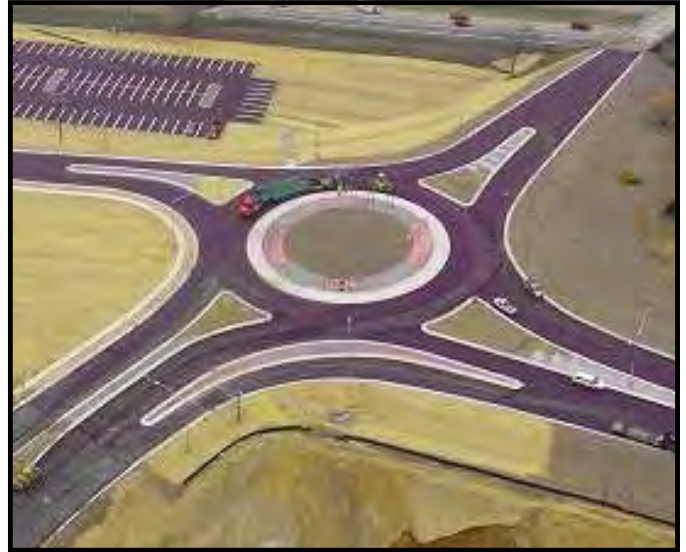
Roundabouts keep traffic moving, decrease emissions, improve fuel economy, and increase safety by slowing traffic speeds and eliminating left turns across opposing traffic lanes. Photo courtesy of the Michigan Department of Transportation.
