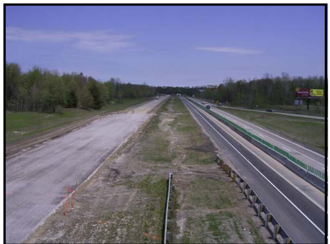
Construction along Interstate 94 at Range Road.
