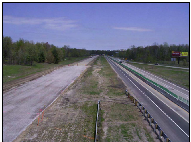
Construction along Interstate 94 at Range Road.
