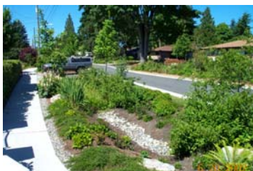
This buffer strip between the home and the street filters and treats stormwater runoff before it enters a storm drain.
