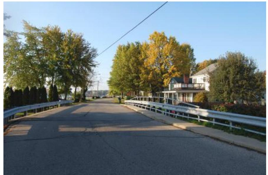
The inadequate approach to the bridge located on Edgewater Street, south of M-29, restricts vertical sight distances and creates a hazard to oncoming traffic.
