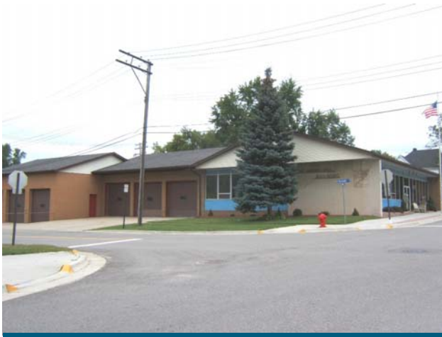
Yale Municipal Building: City Offices, Fire and Police Departments.
