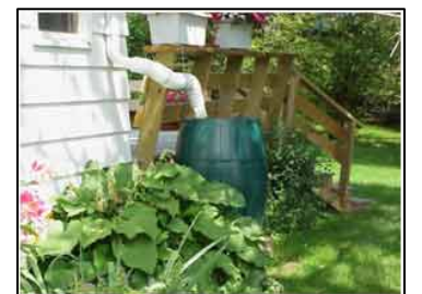
A residential rain barrel collection system.
