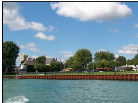
Over 60% of the St. Clair River's "soft" natural shoreline has been "hardened" by the construction of seawalls.
